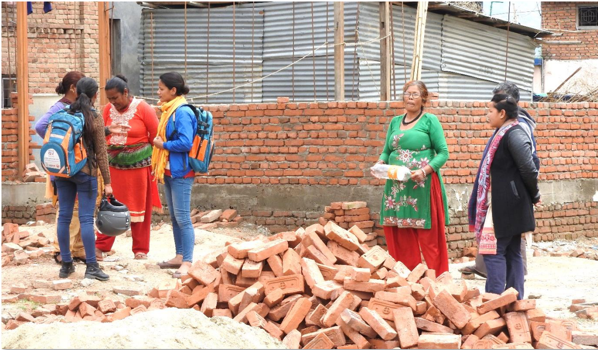
During the mobile clinic at the construction site, Kageshwori Manahara ©NSET
